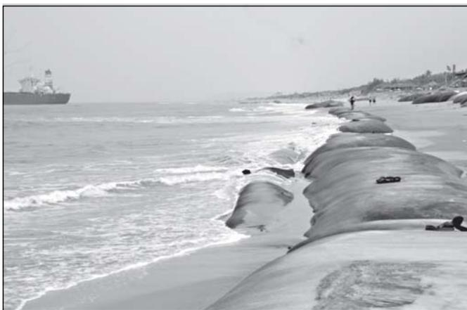
Fig. 5 - Near shore geotextile tubes reef at Candolim beach, Goa (2010)
