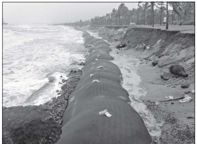
Fig. 4 - Geotextile tubes laid at Candolim beach, Goa (2009)
