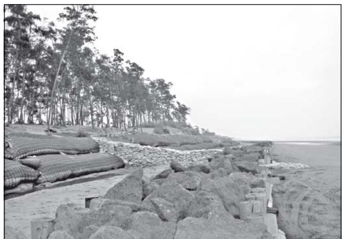
**Fig.3 - Geotextile tubes as a coastal protection at Shankarpur, West Bengal (2008)**
