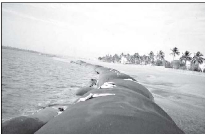
**Fig. 7 - Near shore geotextile tube reef at INS Hamala, Mumbai (2010)**
