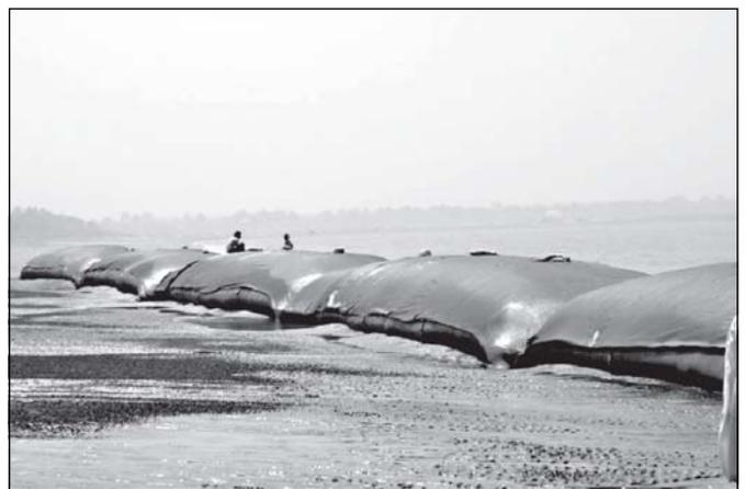
**Fig. 8 - Offshore reef with geotextile tubes at Dahanu, Maharashtra (2011)**
