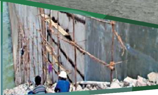
Repairs to upstream face of Almatti Dam Karnataka
